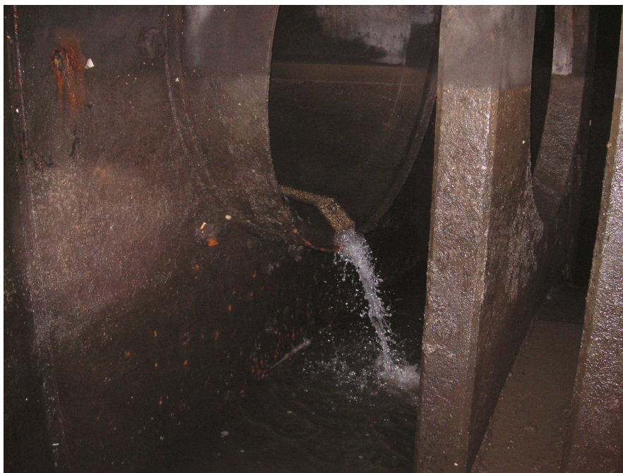
Figure 9. Inlet pipe at the pumping station at Gullbergsmotet. A sample was taken from the free falling flow. (Photo: SGI).
