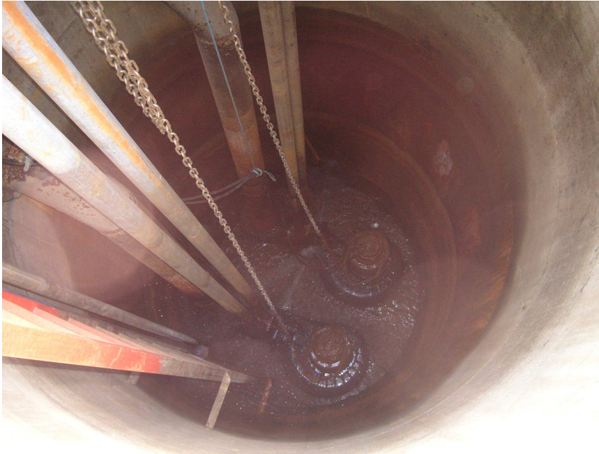
Figure 11. The pumping station at Gullbergsvassgatan (photo: SGI).
