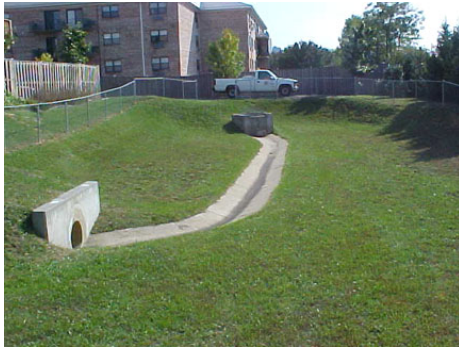
Figure 22 An area that can be used to collect storm water (Courtesy Fairfax County, 2011)
