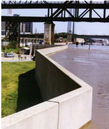
Figure 5 In 1993 in St. Louis District (USA) a concrete wall prevented a flooding of the area, USACE (2011)
