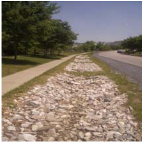
Figure 18 Infiltrating ditch (Sustainable Storm water Management, 2010).
