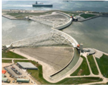
Figure 2 Maeslantbarrier at Rotterdam (Delta Marine Consultants, 2010)
