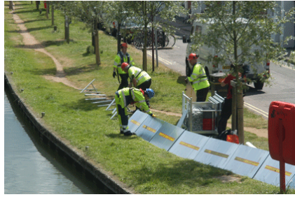
Figure 8 Temporary pallets (Geodesign AB, 2010)
