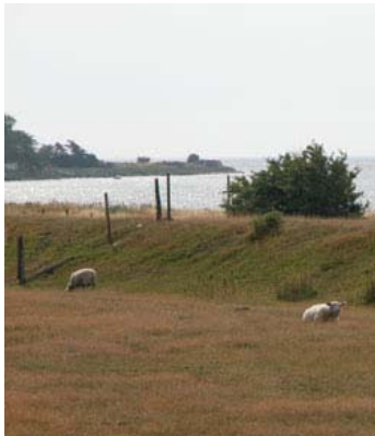
Figure 4 Soil embankment (Trelleborg Municipality, 2010)
