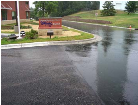
Figur 16 Permeable asphalt (Ramsey-Washington Metro Watershed District, 2011)
