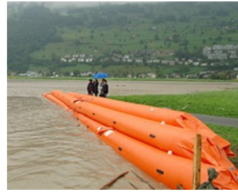
Figure 9 Tube wall with air bags (Geoline Ltd. 2011)
