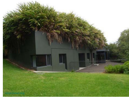
Figure 25 Green roof in Sydney (Water Sensitive Urban Design, 2011)
