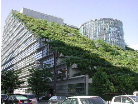
Figure 24 Green roof (Scholtens Roofing, 2010)
