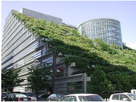
Figur 26 Grönt tak (Scholtens Roofing, 2010)
