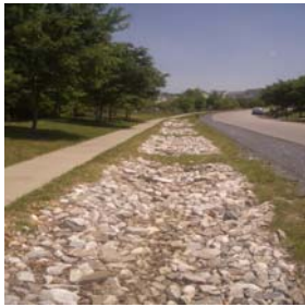
Figur 20 Infiltrerande dike (Sustainable Stormwater Management, 2010)
