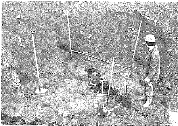
Fig. 3. Location of the sand drains after removal of the gravel fill.
