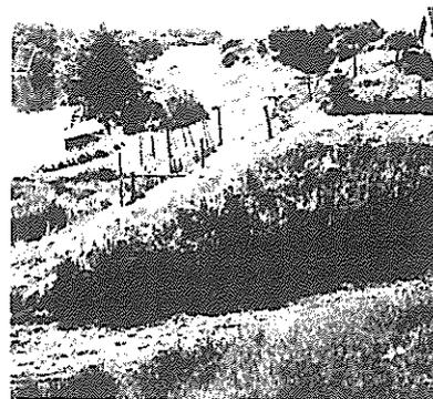
13. Increase of slope stability by excavation at top of slope.
