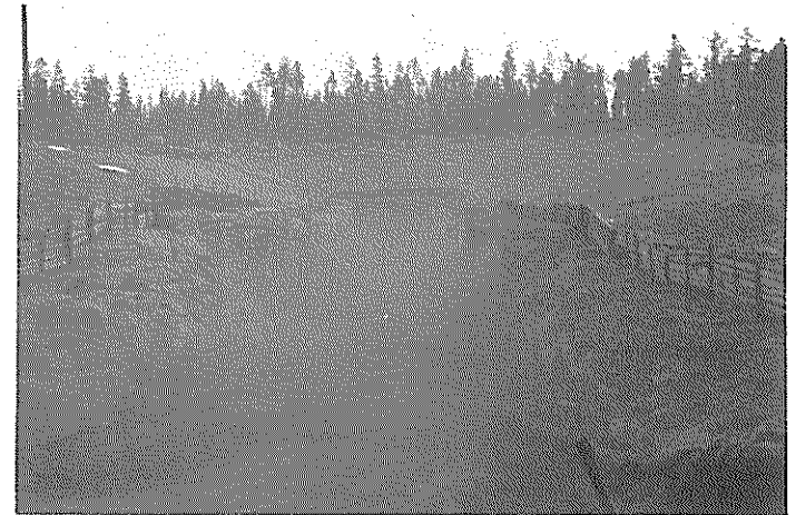
(c) Extremely Poor Visibility. Tunneling operations halted.
