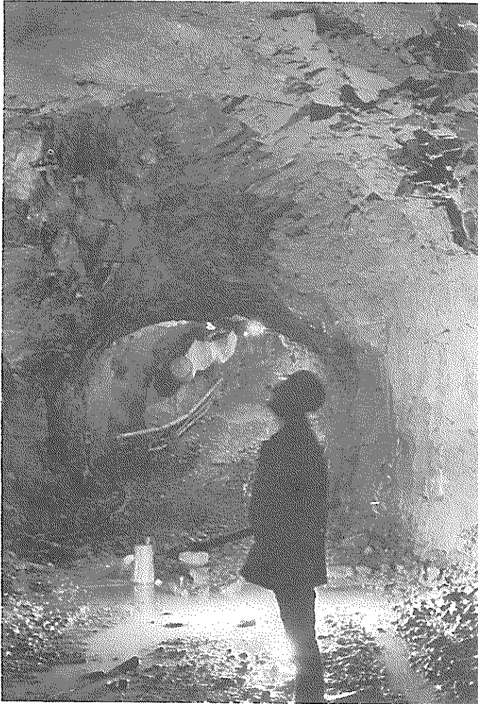
Fig. 2.13 Case 37. Access tunnel at Vietas. Example of progressive roof falls in heavily fractured rock; formation of vault- or dome-shaped opening; support necessary to stop loosening; fallout exceeds one-half of tunnel area
