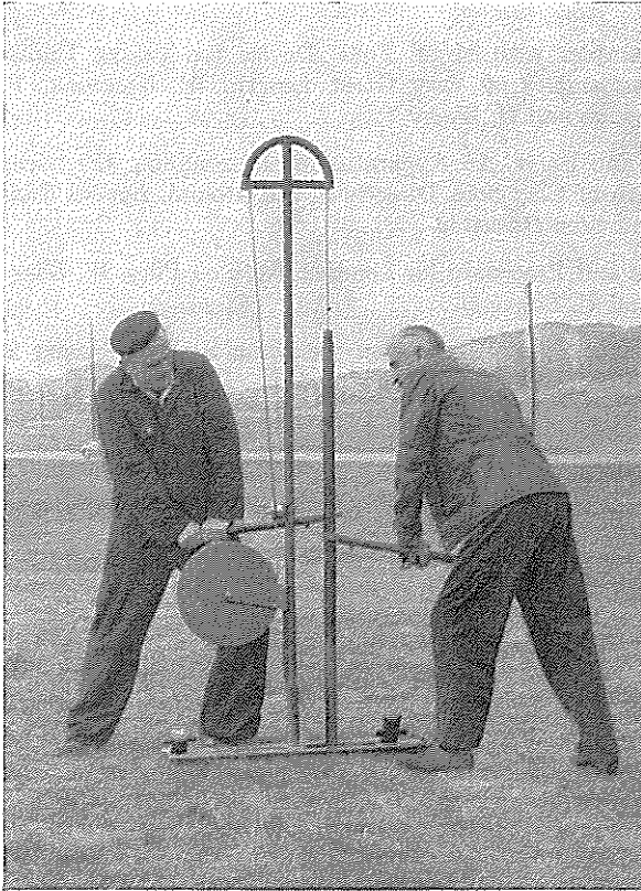
Fig. 21. Standard sampler during punching.
