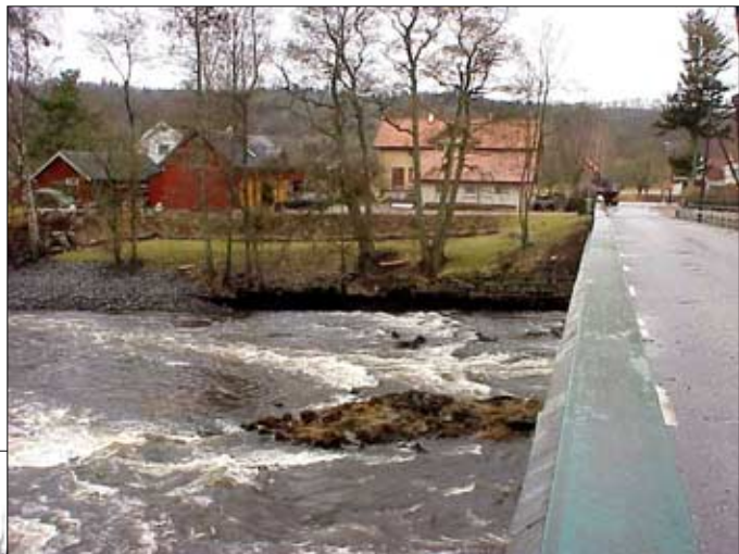
b) The bridge seen from the east with the torrent and erosion protection downstream.
