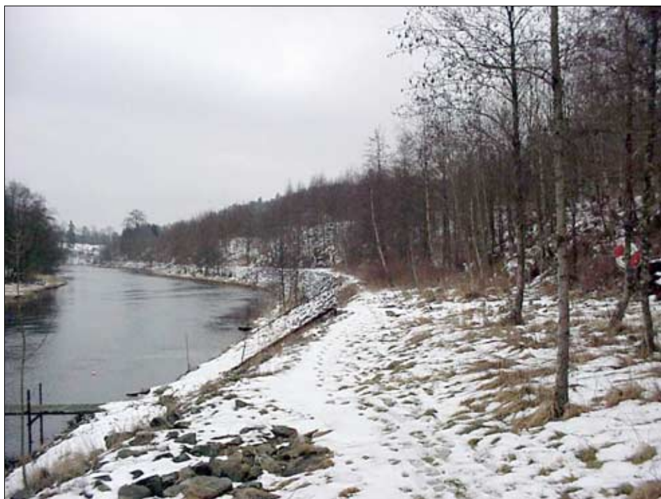
Fig. 5. View of the eastern slope towards the river and its erosion protection.
