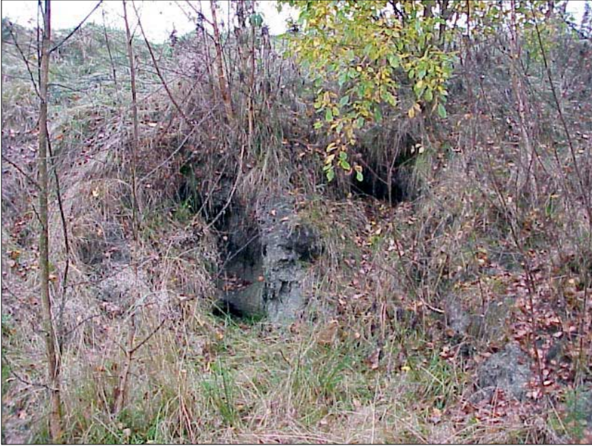
Fig. 83. Example of internal erosion in sand and silt in the upper slope.
