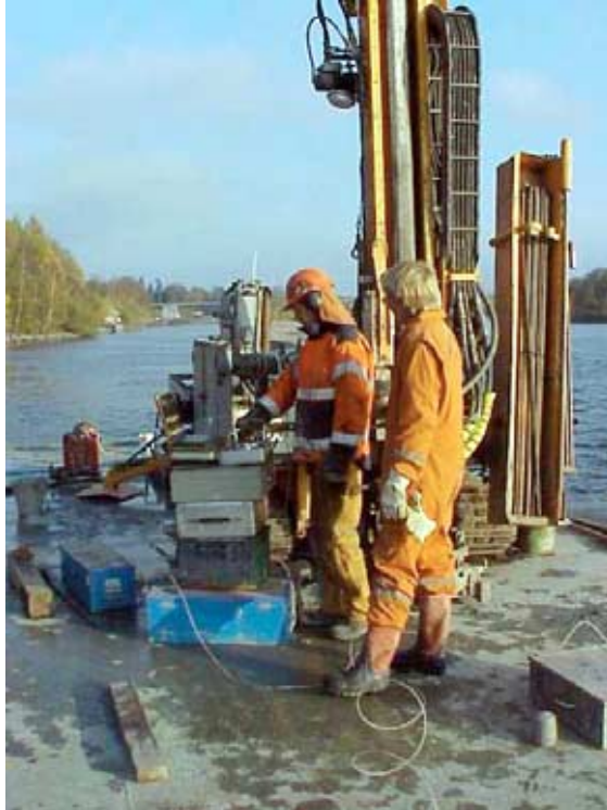
Fig. 87. The raft and drill rig in position in Point I out in the river. b) Preparations for a dilatometer test with automatic recording of test data in point I. The bridge at Lilla Edet and the entrance to the lock at Ström can be seen in the background to the left of the drill rig.
