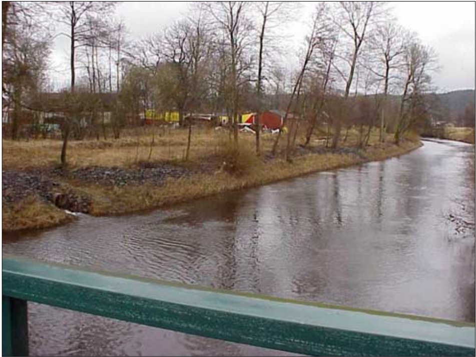
Fig. 134. Erosion protection and excavated area on the west side of the river north of the bridge.
