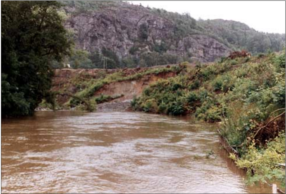
Fig. 2. Ongoing erosion and small slides before construction of the erosion protection.
