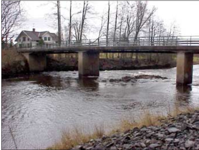
a) The bridge seen from the north with the barrier of stone blocks.
