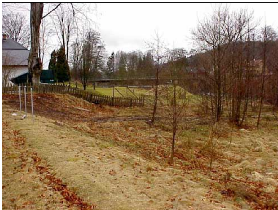
Fig. 135. The northernmost part of the excavated area with the lawn in front of the nursing home in the background. The tracks of the crawler drill rig can be seen on the ground surface with free water standing in them.
