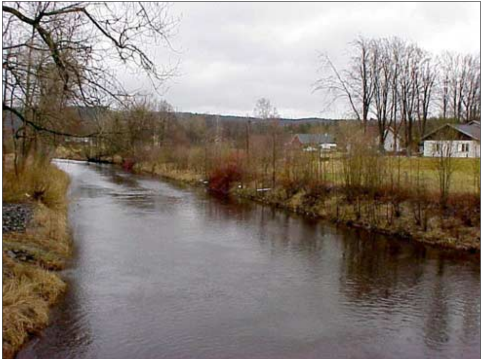
Fig. 122. The river Viskan to the north of the bridge in Sundholmen. The white plastic tubes that protrude from the slope are parts of the drainage system for the excavated terrace behind.
