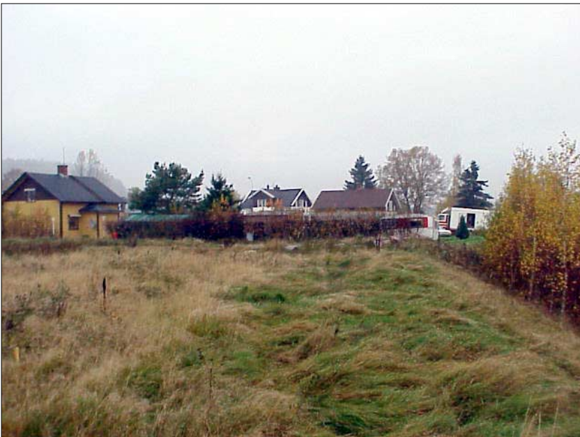
Fig. 84. The crest of the upper slope and remaining buildings. The truck in the background is partly backed down on the access road to the excavated terrace.
