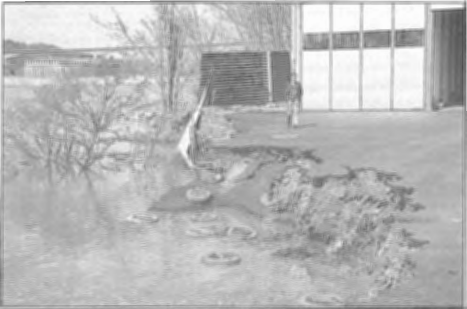
Figure 1. The landslide at Agnesberg, 14 April 1993, came very close to an existing industrial building. (Photo by Sven Liedberg, CTH)
