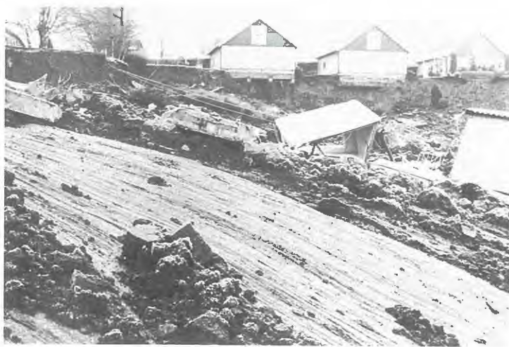
Slip surfaces close to firm bottom in the upper part of the slide area.
