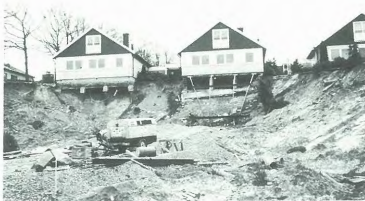
Temporary support for houses.
