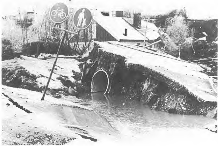
Demolished houses and broken up ground in the slide area.
