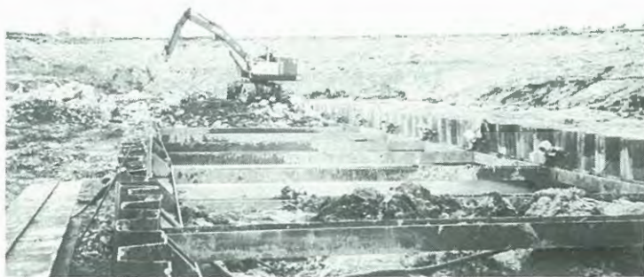
Placing of rockfill between back tied sheet walls
